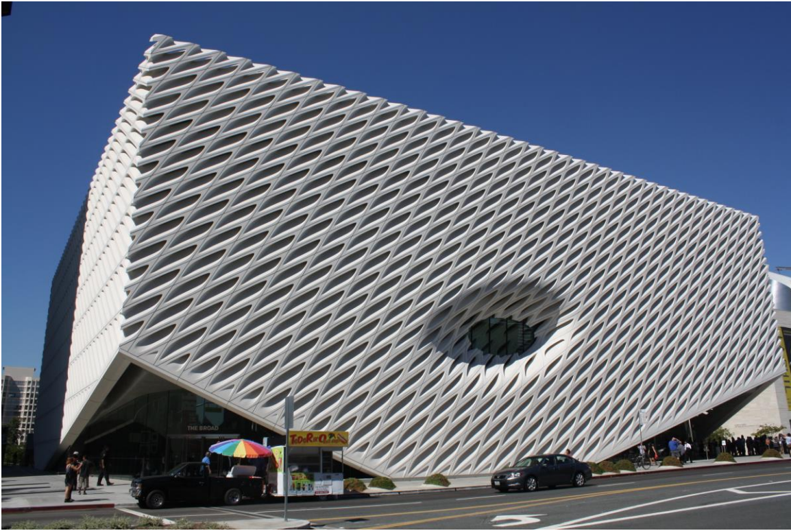
GFRP lightweight concrete cladding panels provide an attractive dynamic exterior cladding to The Broad Museum in LA.
